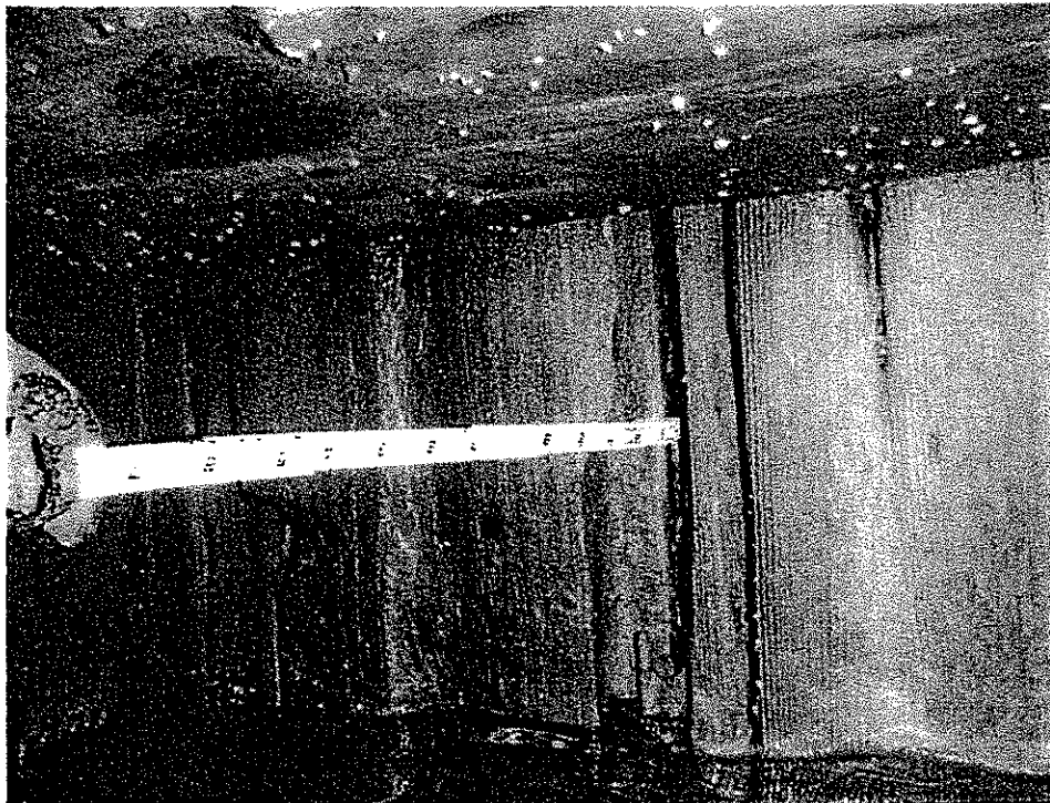
PHOTO 8. General view of deterioration in timber sheet pile bulkhead. Note penetration with the ruler exposing voids behind the bulkhead.
