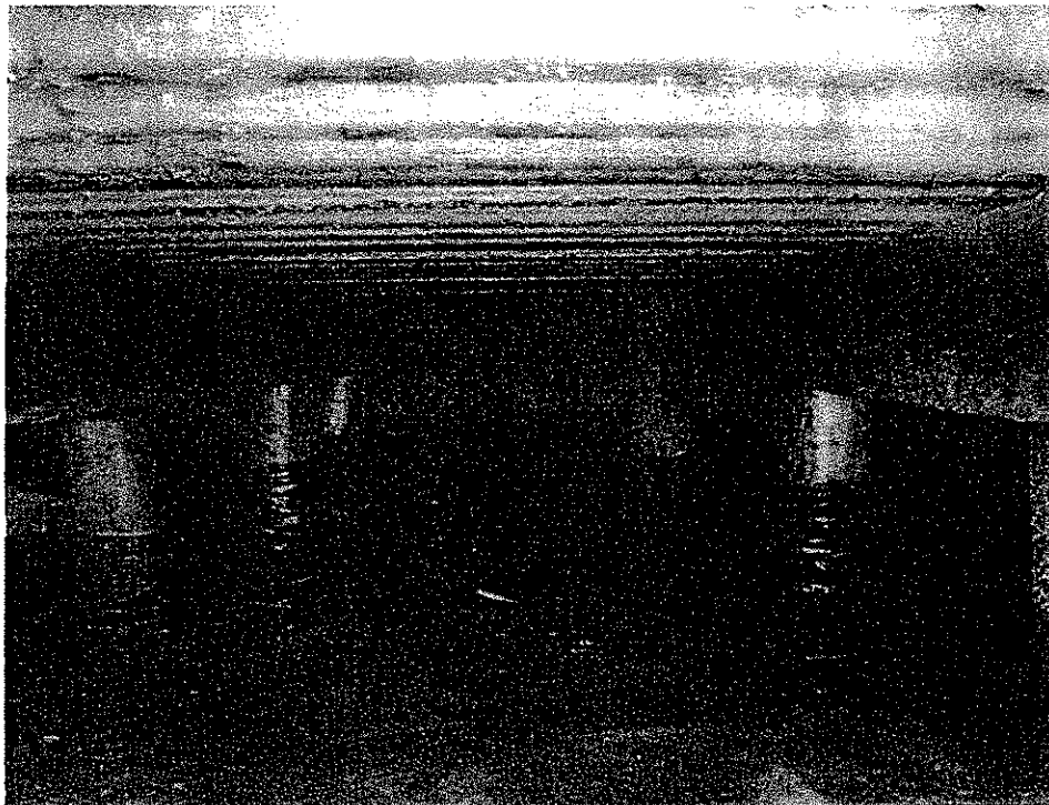
PHOTO 12. General view of corrugated steel deck with moderate deterioration.
