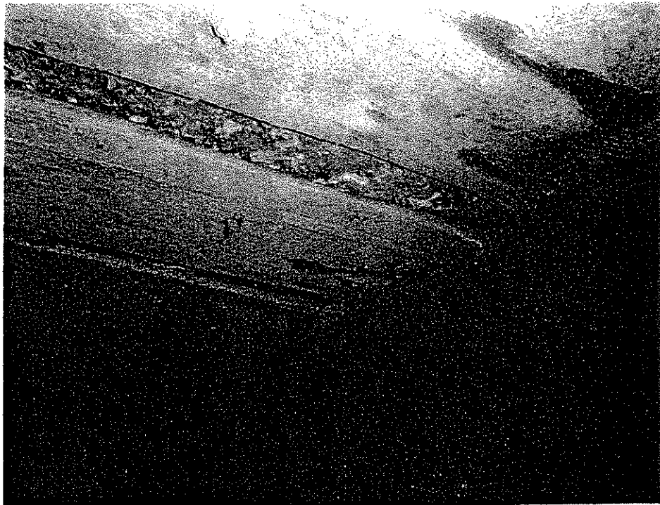
PHOTO 4. General view of deterioration in timber deck exposing concrete structural deck.
