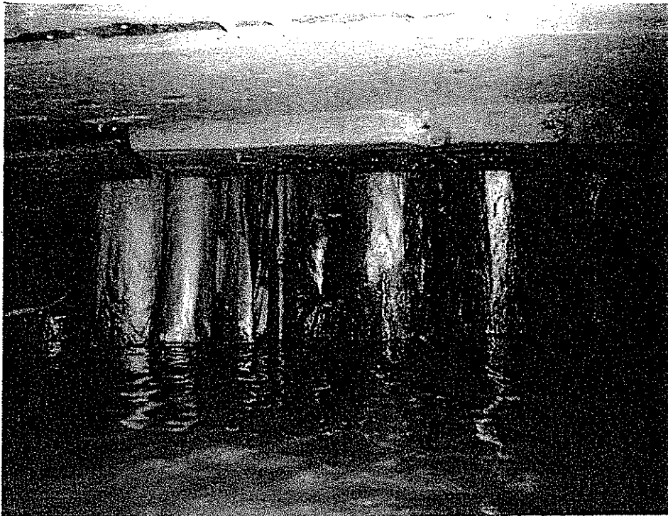
PHOTO 5. General view of deterioration in timber soldier pile bulkhead. Note gaps and rot in the timber piles.
